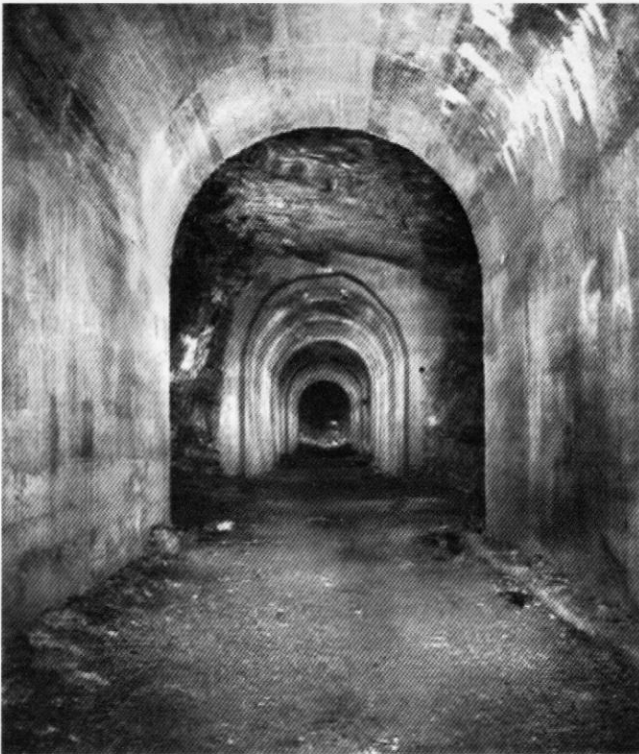
The main tunnel at Ho2 in 2003.
